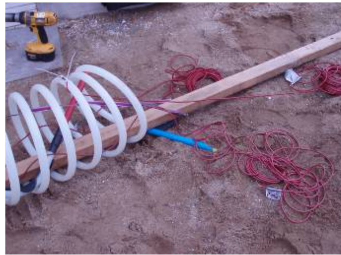
E. Helix Probe with 3no wires that connect to Sensors
