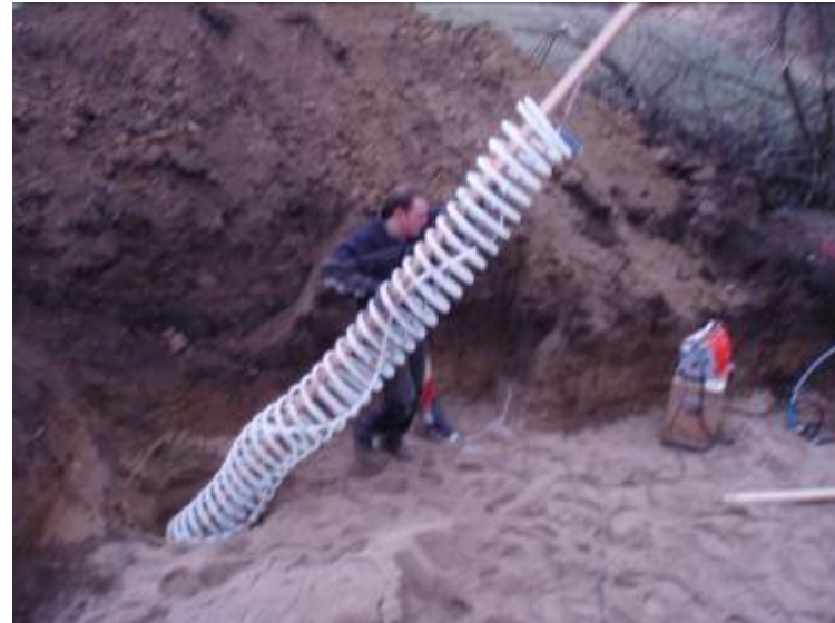
D. Helix Probe with Sensor
