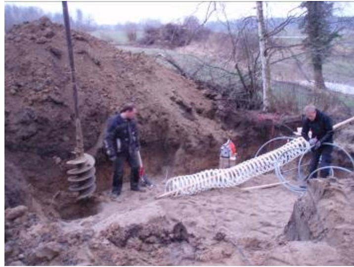
E. Helix Probe with 3no wires that connect to Sensors
